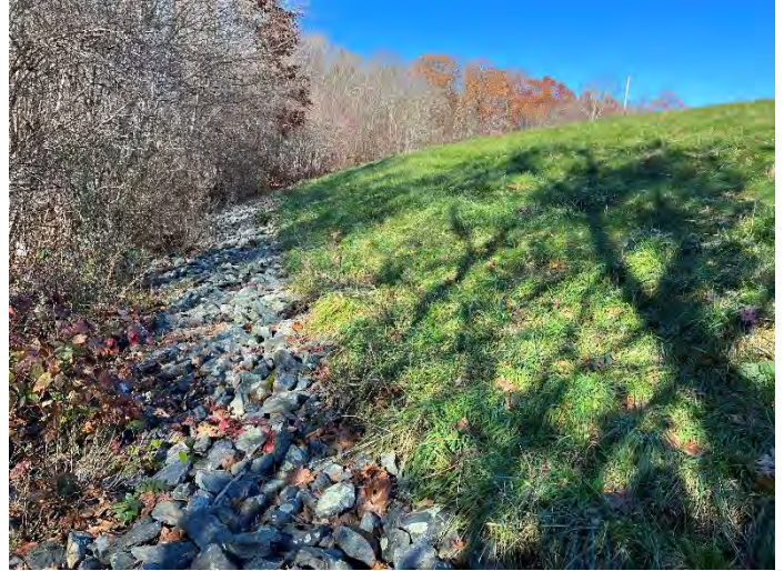
Photograph #22 Toe of slope rip rap protection.
