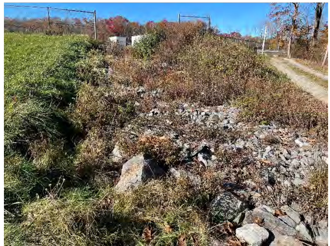
Photograph #8 Rip rap outlet from Basin 2 and weir.
