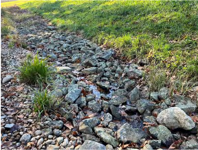
Photograph #21 Toe of slope rip rap protection.
