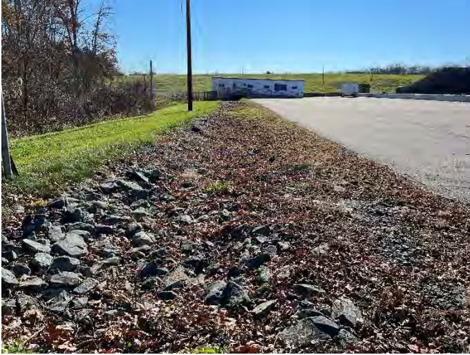
Photograph #13 Rip rap swale on east side of transfer station and edge of pavement cap functioning and in good condition.
