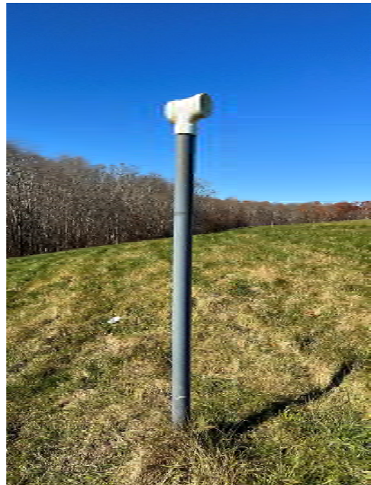
Photograph #24 Gas vents in good condition.
