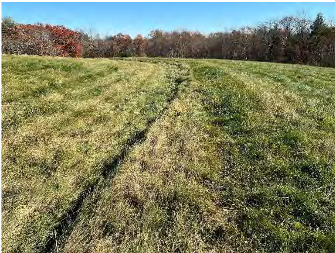
Photograph #11 Grass swales in good condition.
