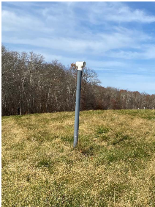
Photograph #23 Gas vent.
