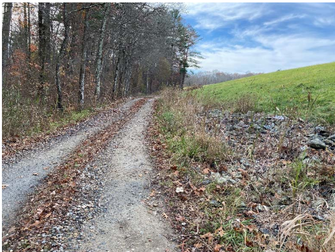
Photograph #3 Eastern gravel perimeter access road.
