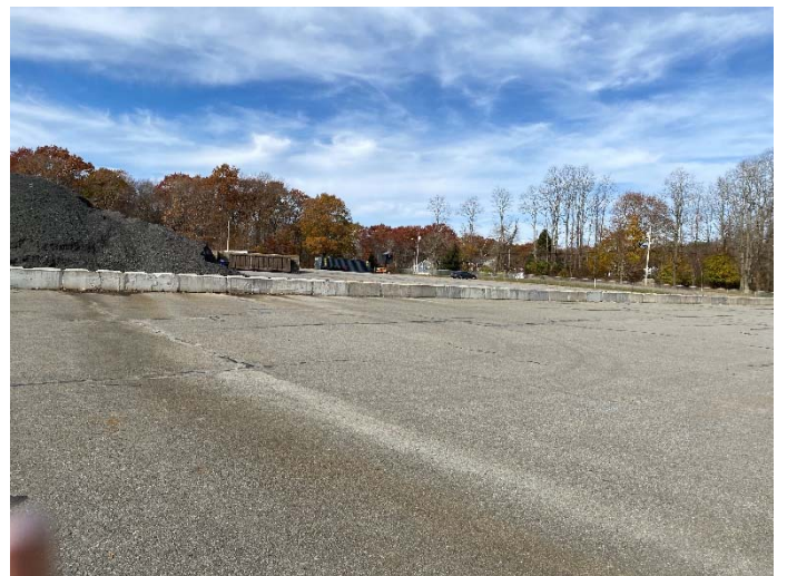
Photograph #4 Pavement cap and transfer station area.
