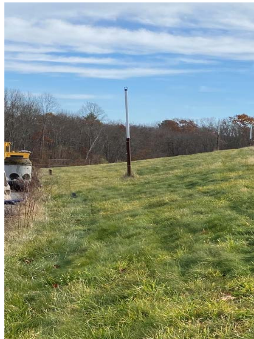
Photograph #24 Gas vents in good condition.
