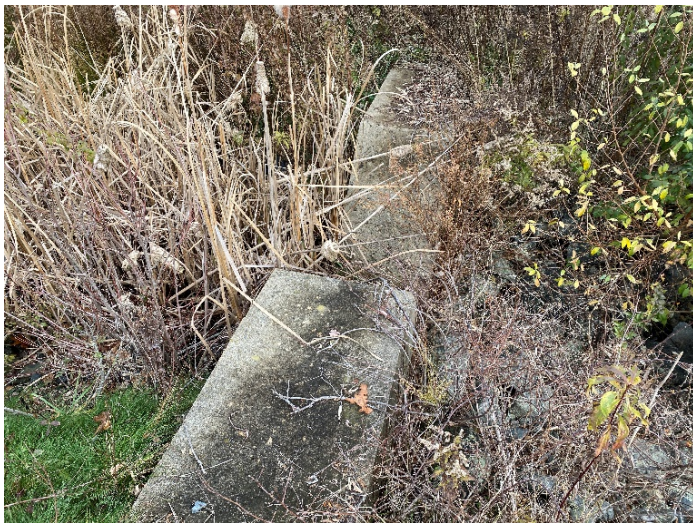
Photograph #7 V-notch weir at outlet from Basin 2.
