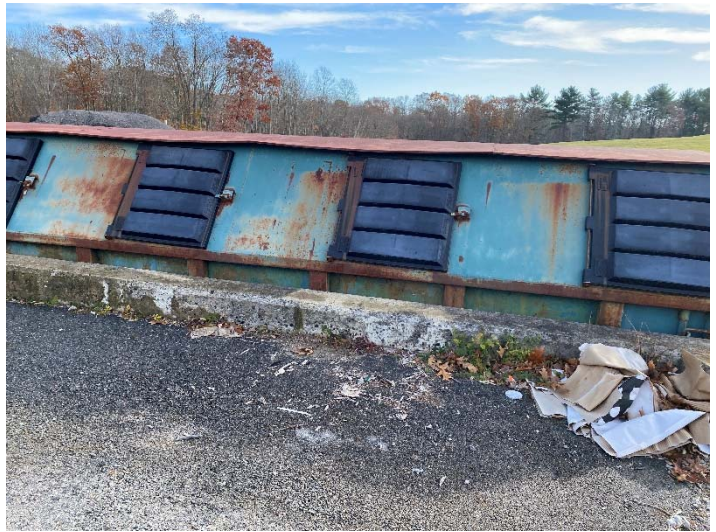
Photograph #22 Commingled recyclables containers.
