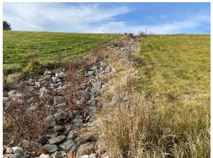
Photograph #12 Rip rap downchute to Basin 1 is in good condition.
