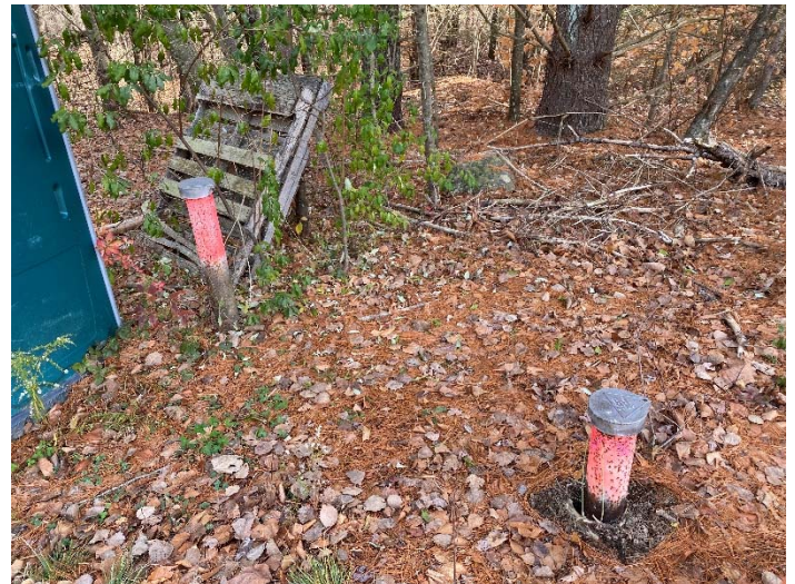
Photograph #28 Groundwater monitoring wells MW-8S and MW-8D in good condition.
