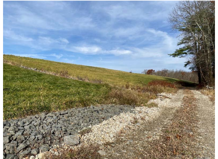
Photograph #16 Eastern slope.
