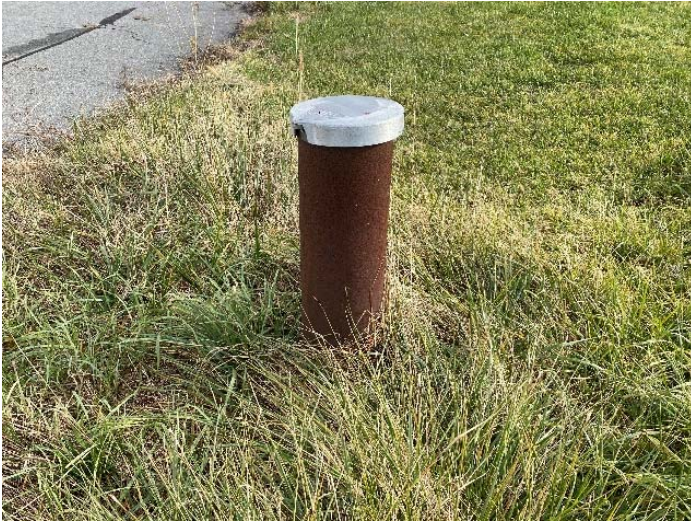
Photograph #25 Gas monitoring well GM-1.
