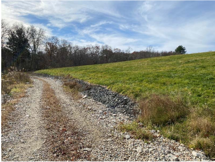
Photograph #21 Toe of slope rip rap protection.
