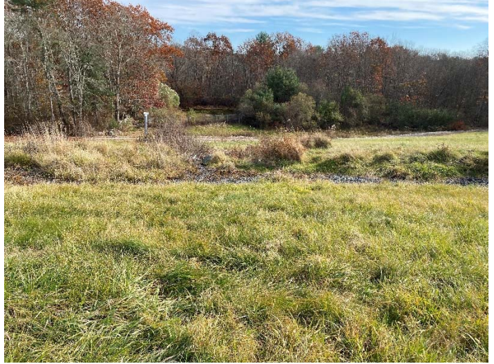
Photograph #14 Stone-lined swale in good condition.
