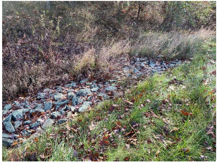
Photograph #22 Toe of slope rip rap protection.
